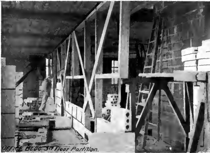
Fig. 3.—Hollow tile floor and partition construction.
